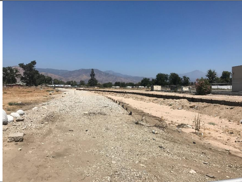
Photo 6. City of Highland West —West Storm Drain channel
